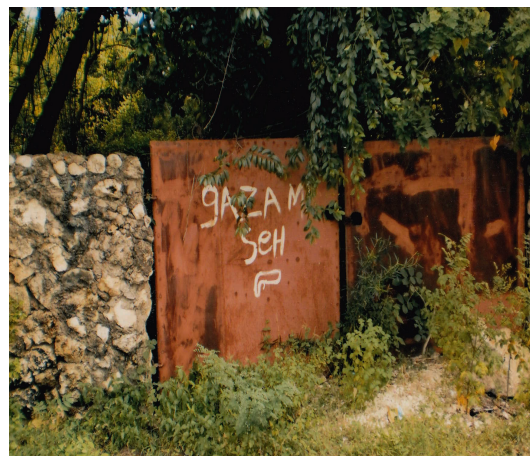
PROPERTY ROAD SIDE WALL AND GATE
